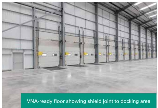
VNA-ready floor showing shield joint to docking area
